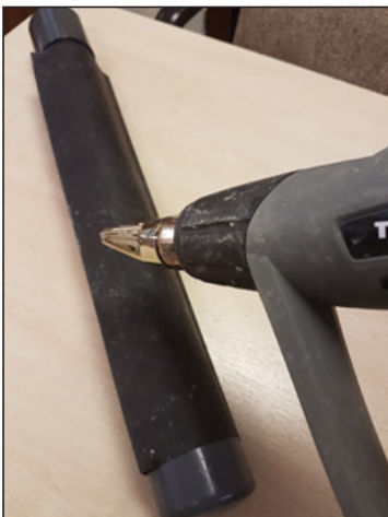
1b. Heat the heat shrink so it is tight on the lateral
