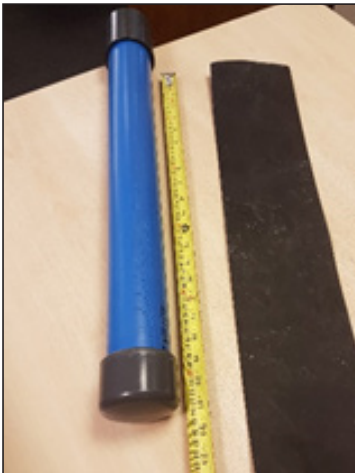
1a. Cut the heat shrink to size
